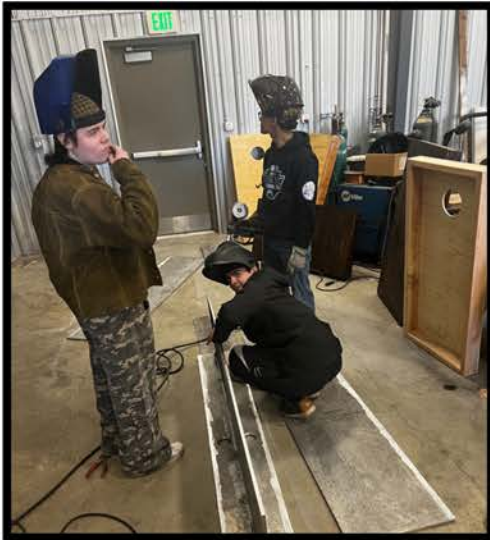
Students are welding a metal box together for the Tonasket Fire Department.
